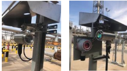
Figure 6. Open path laser gas detector (ELDS) transmitter (left) and receiver (right)
