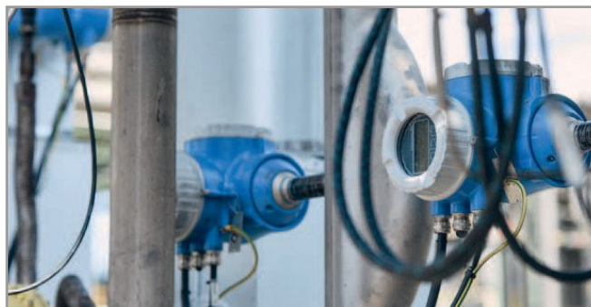
Figure 1. For specialty chemical manufacturers, Coriolis mass flowmeters with self-diagnostic technology support in situ testing and verification. (Shown: Promass F 300 with Heartbeat Technology)
