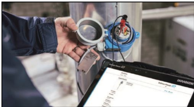
Figure 4. For an acrylics-based products manufacturer, a configurator tablet creates a mobile field workstation, enabling diagnostic work without interrupting a process. (Shown: SMT70 Field Xpert)
