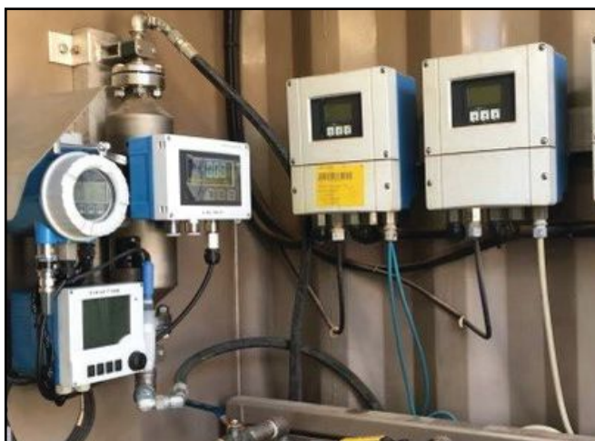
Figure 3. Coriolis flowmeters handle the viscosity fluctuations of nitrogen processes and can wirelessly transmit multiple process values and instrument diagnostic data via HART, WirelessHART, and Bluetooth. (Shown: Proline Promass I 300)
