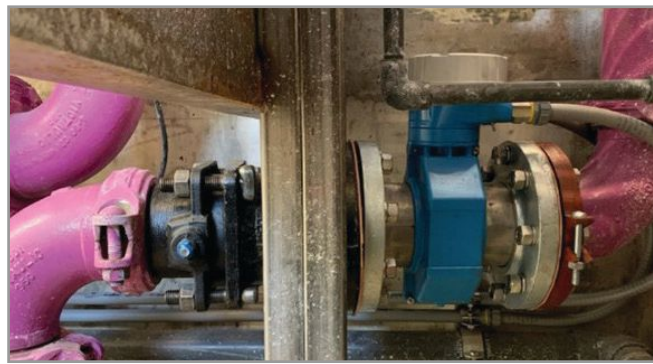
Figure 5. Smart electromagnetic flowmeters enable flow measurement in tight spaces, such as those found in water treatment plants. (Shown: Proline Promag W 400)
