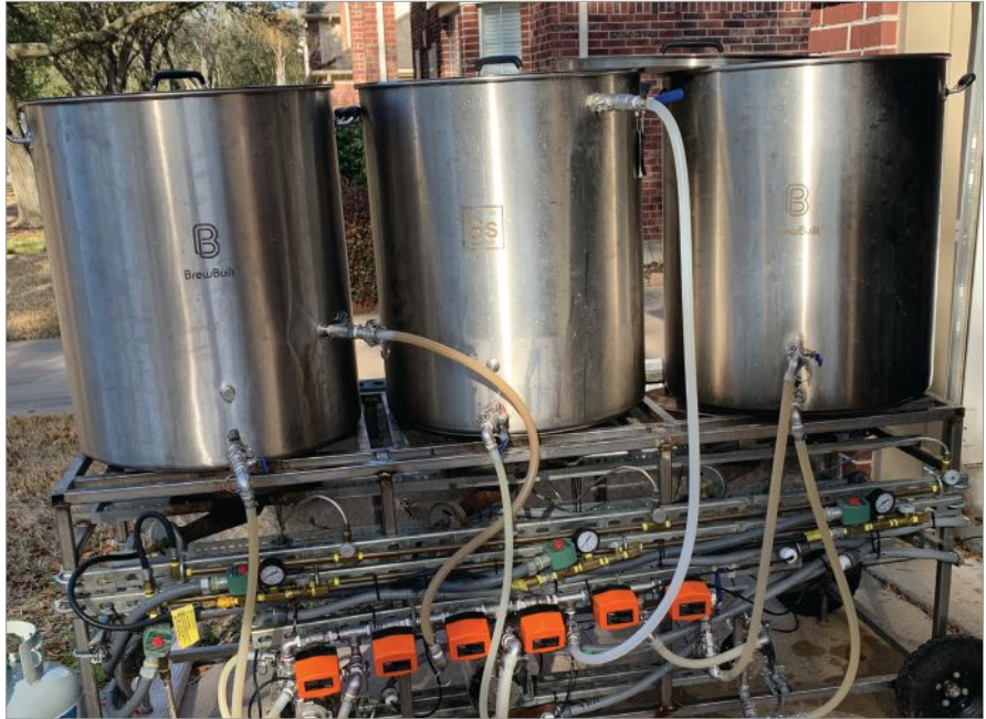
Figure 1. This homebrew rig started as a completely manual operation but is now monitored and controlled by an AutomationDirect CLICK PLC, level sensors, solenoids, and more. Its operation can be viewed and controlled remotely with a smartphone.
