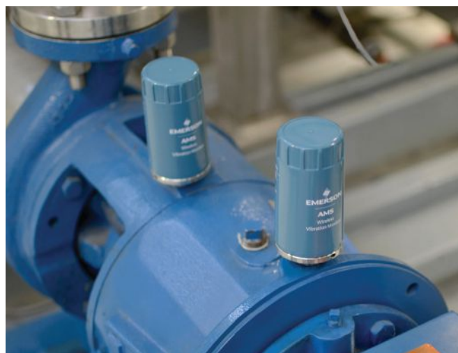
Figure 2. Small wireless sensors, like the Emerson AMS Wireless Vibration Monitors shown here, are simple to install, making it easy to monitor plant assets.
