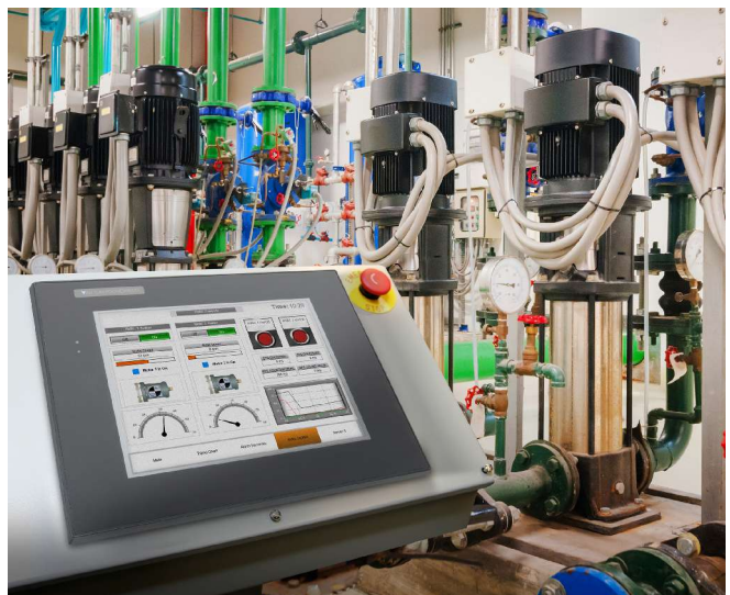
Figure 4. HMI remote app: A dedicated HMI can provide local control as well as remote access at a reasonable cost.
