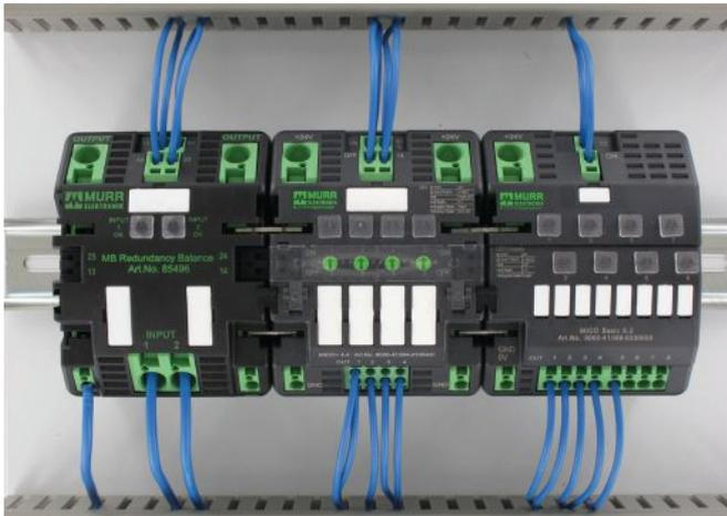
Figure 2. Individual ECP modules, like the three devices from the Murrelektronik MICO line shown here, enable bulk 24 VDC control panel power to be distributed to one, two, four, or eight individual Class 2 circuits.
