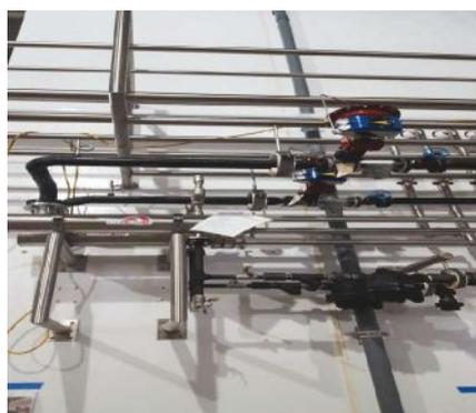
Figure 4. The cheese manufacturing plant after implementing a rotary control valve and other best practices.
