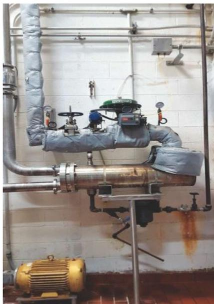
Figure 3. A Midwestern cheese manufacturing plant “before,” using an automated ball valve and a range of improper practices.
